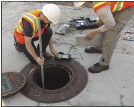
Figure 1. Ultrasonic Thickness Testing Implementation
